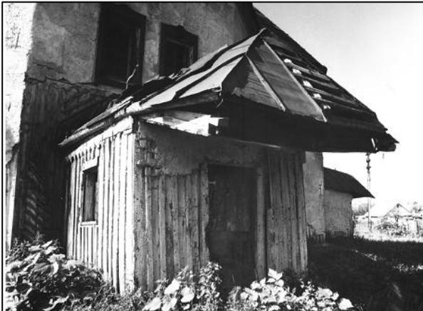
The exploitation of church as a storehouse leads to the destruction of the lower beam level. The lack of ventilation and premises' aeration lead to the appearance of mould. Later on the fungus spreaded over the entire surface of the walls and the wooden floor.
