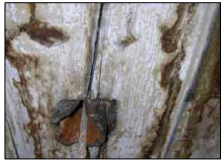
13. Water leaking over the wooden wall frame, Church Albrechtice
