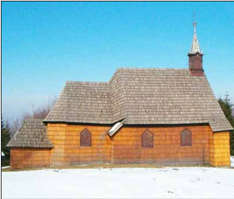
17. The present church is shown in the figure. It has a single-nave gothic structure with polygonal presbytery and rectangular sacristy and a late gothic roof structure.
