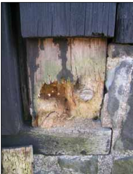
15. Wood degradation by brown rot fungi, Church Albrechtice
