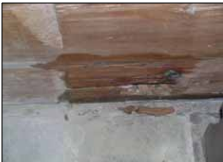
13. Water leaking over the wooden wall frame, Church Albrechtice
