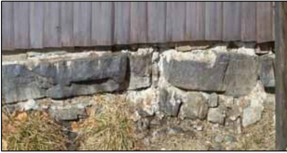
19. Socle of free-laid stones, recently sealed with cement grout.
