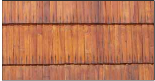
20. Timber walls of hewn timber or round logs covered with shingles.
