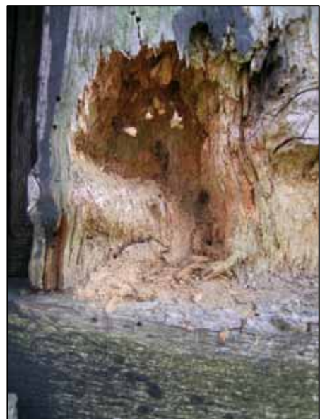
15. Wood degradation by brown rot fungi, Church Albrechtice
